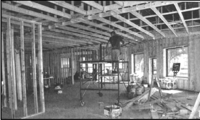
Sand County Contractors at Work
