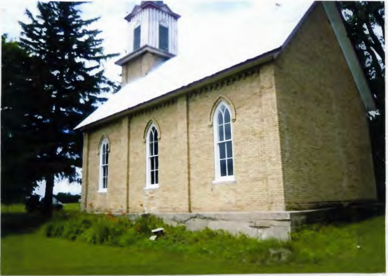
The South side of the Westfield Church, showing the condition of the original brick walls and the window treatments.
