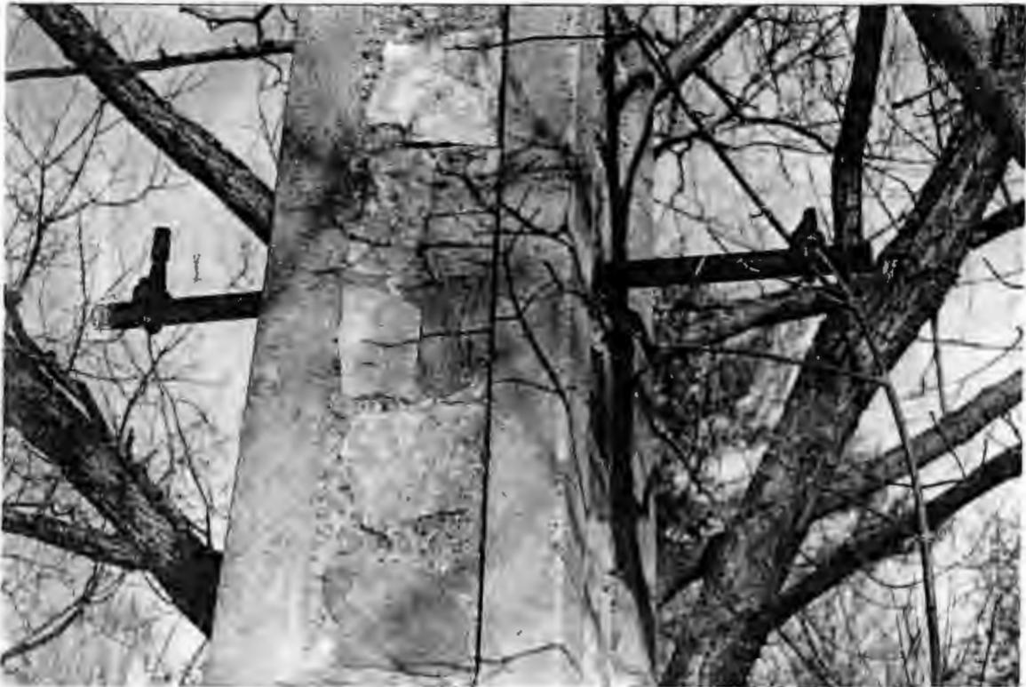
This photo of a portion of the historic obelisk shows the unusual construction, with imbedded quartzite stones and steel cross-arms for the electric power insulators.
