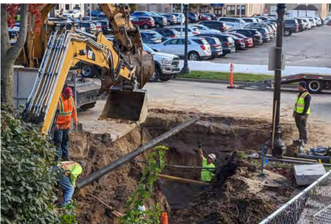
Installing the new water line
