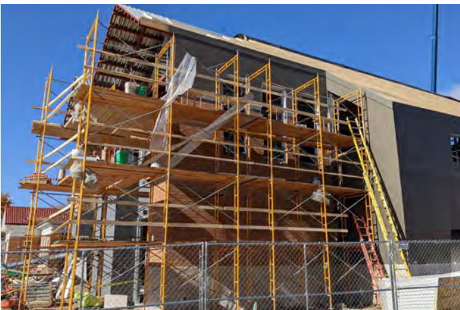
Scaffolding and newly laid bricks on the walls
