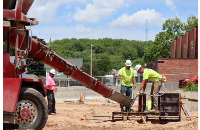
Pouring cement foundation footings.
