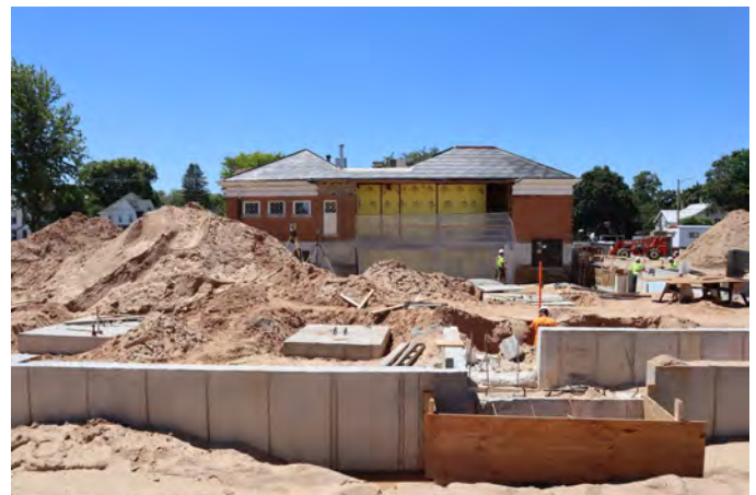
East addition cement foundation footings.
