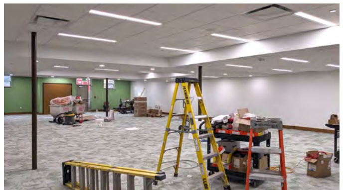
Lower level of the Carnegie building
