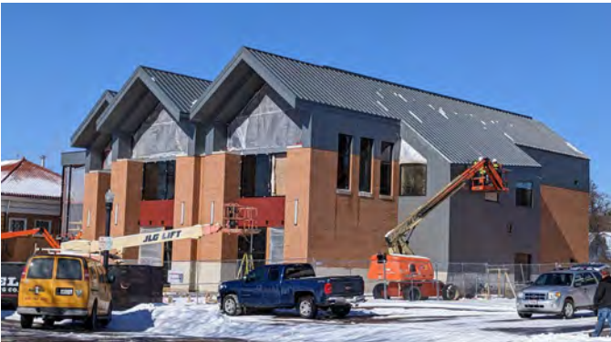
Working on the siding
